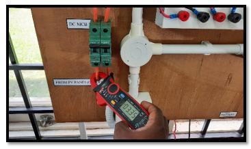
Figure 1. Photovoltaic current measurement
